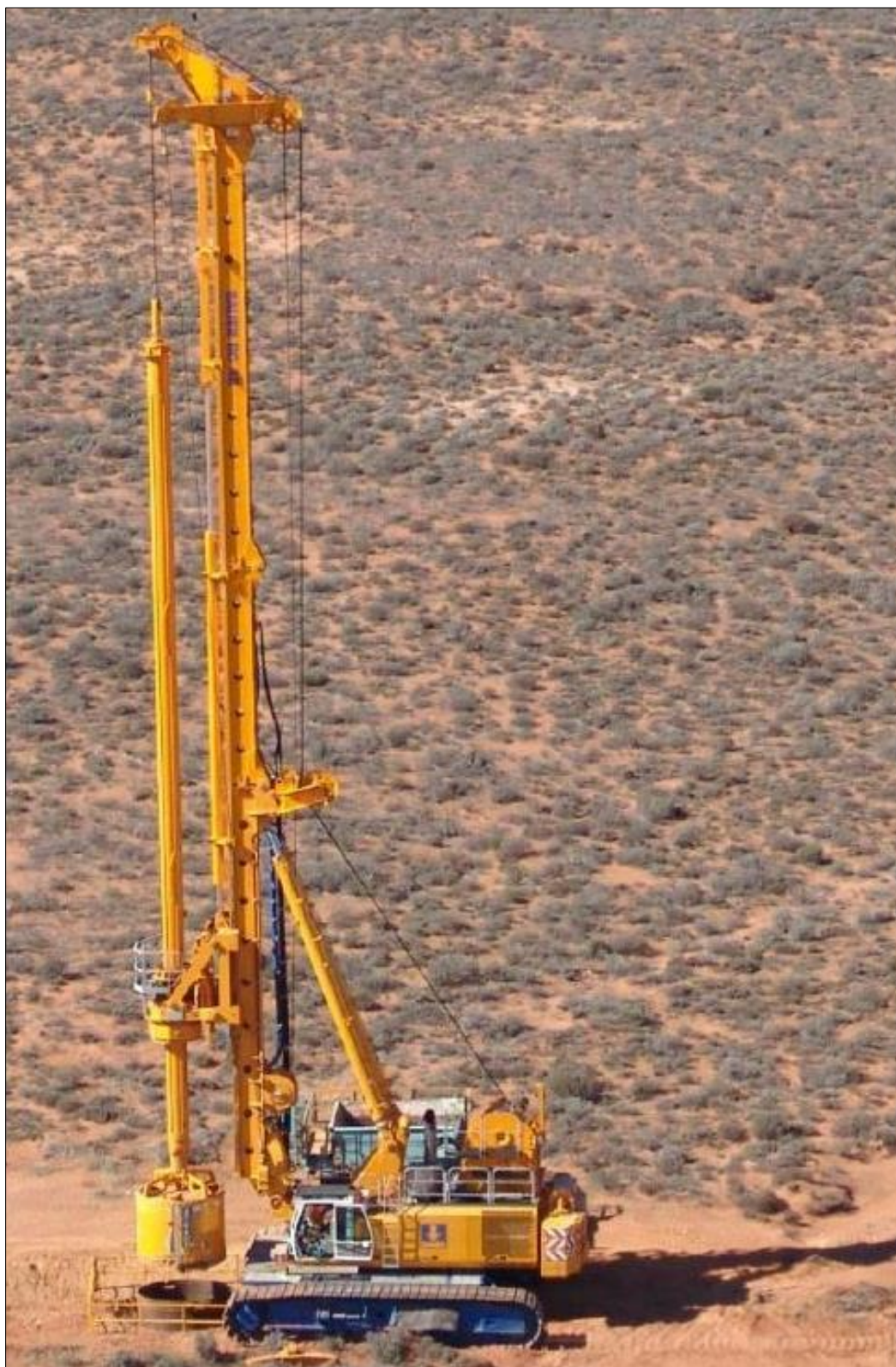
Figure 7 Bauer BG48 rig drilling with 2,400 mm bucket in South Africa
